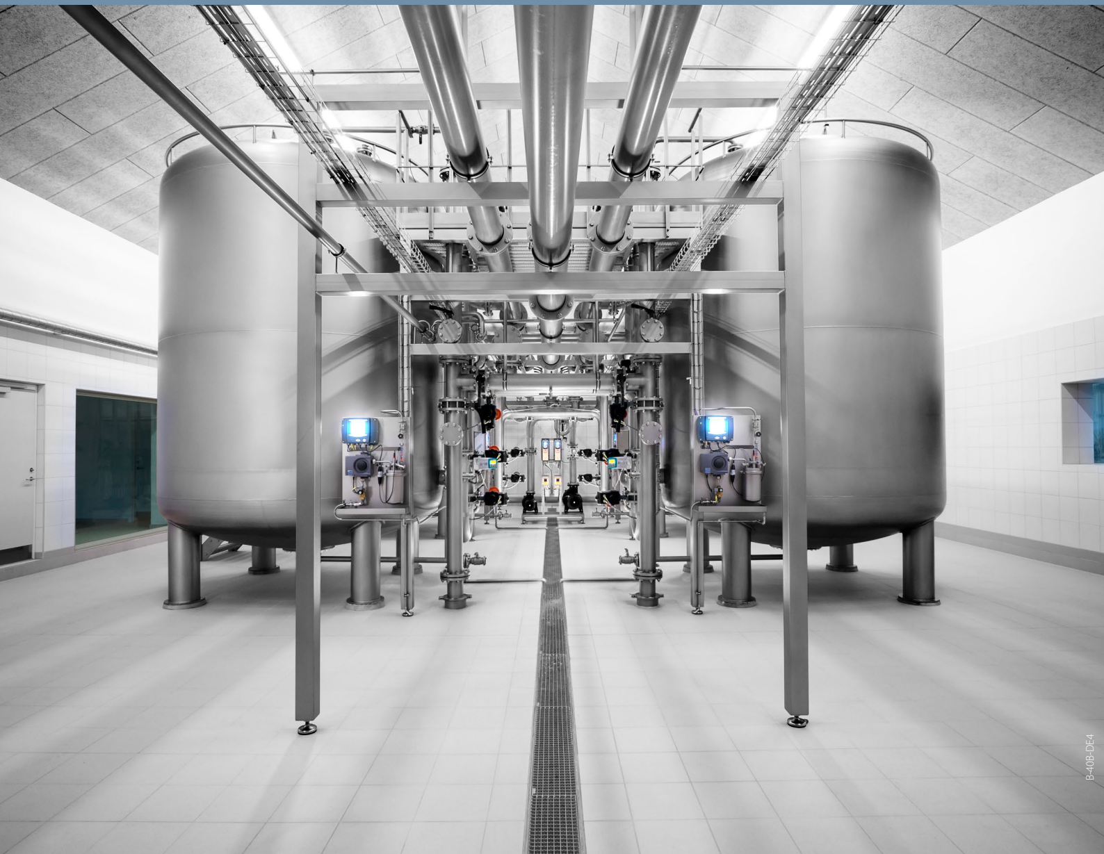
Reduction of iron and manganese at a waterworks in Denmark. The cutting edge technologies used for online measurements, oxygenation and pressure filtration helps secure the supply and drinking water safety. The solution comprises 4 x TFB 100 units with a shell height of three meters arranged in two parallel production lines. The flow rate is up to 270 m 3 /h.
